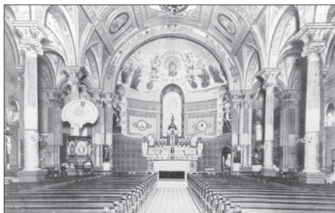
The earliest photo of the interior of the present church, shows the central window in the apse directly behind the altar before the installation of the Great Mosaic in the 1920's. That window, St. Francis in Glory, can now be seen in the 31st Street vestibule of the church.
